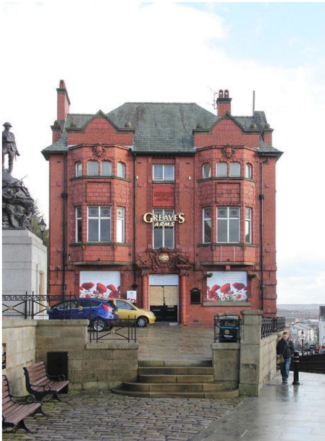
Fig.57 Greaves Arms P.H., Yorkshire Street, Oldham.
