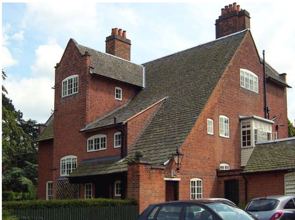
Plate 17 1892 Inglewood, Leicester: A rare work by Ernest Gimson who worked alongside Henry Wilson in Sedding's office. Photo: NotFromUtrecht, Creative Commons Attribution-Share Alike 3.0
