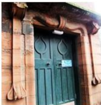
Fig.25 Credit: Gerald Blaikie
