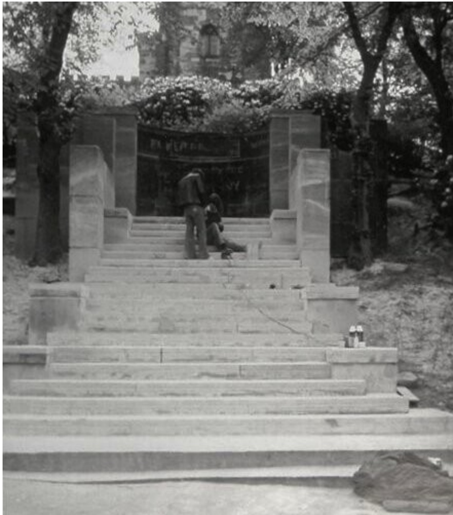
Illustration 17: Sandblasting and removing nosings 1978. Trees abut. (Photo: Middleton Library)
